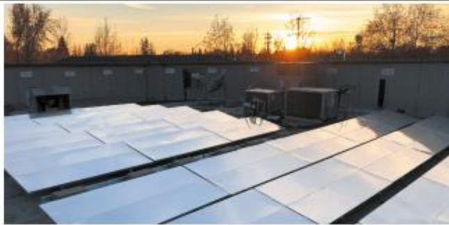
Super-cool panels on the roof of a shop in Sacramento, California.
